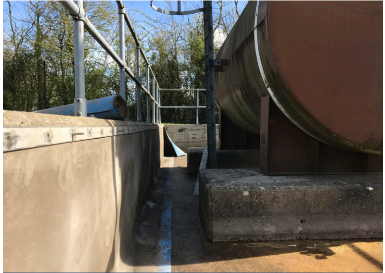
The CCH5™ was hung vertically using steel clamping bars
