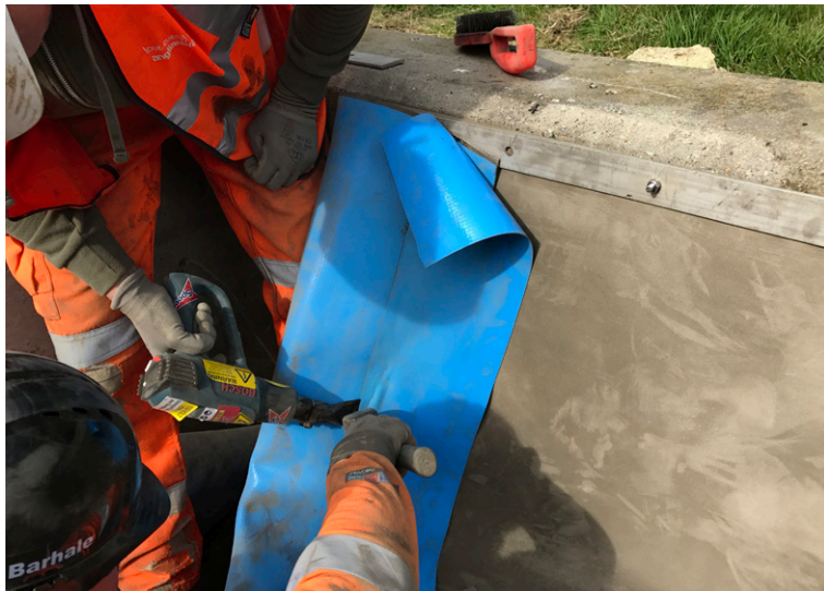
Additional PVC for corner details were welded with a heat gun
