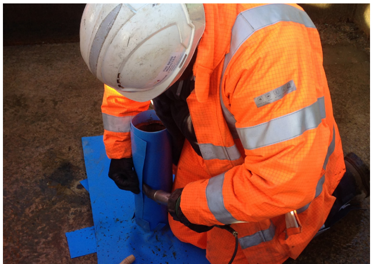
Upstands/terminations were hand-welded
