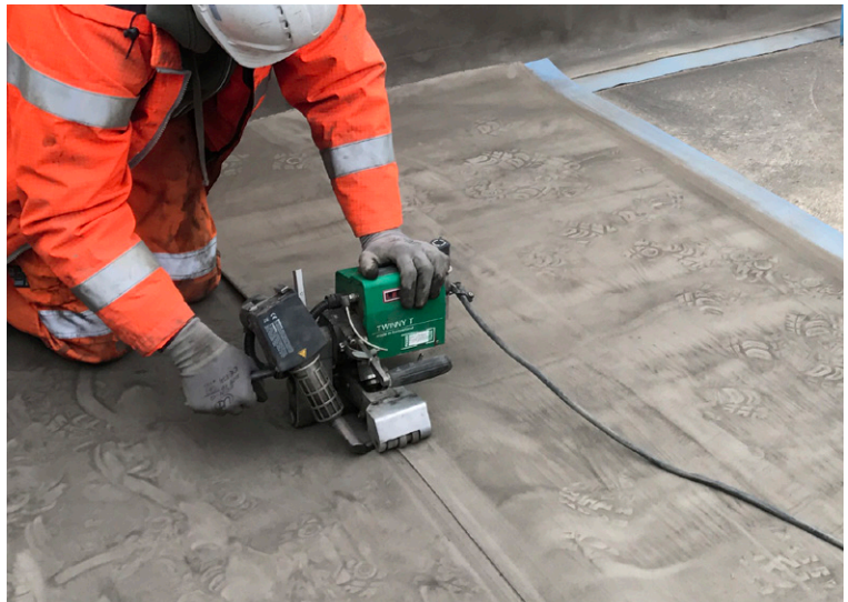
Joints were triple track welded where possible
